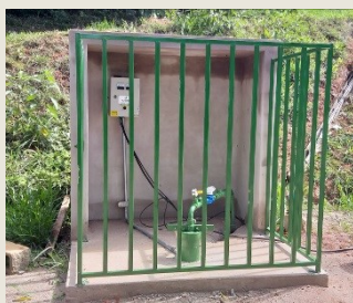
Security gate made for a well
