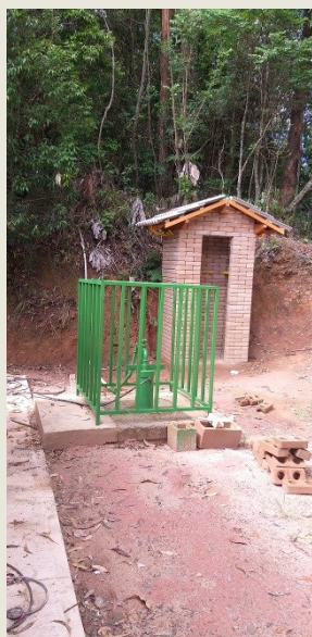
Utility box made from homemade bricks & new pump gate
